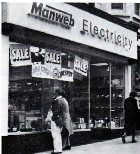
The neat fascia and inviting entrance to our new shop at Colwyn Bay.
